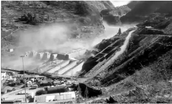
Figure 1: The Tapovan Vishnugad power plant — a 520 MW run-of-river project constructed on Dhauliganaga River in Chamoli District of Uttarakhand was hit by a massive glacial debris flow on 7 February 2021.
