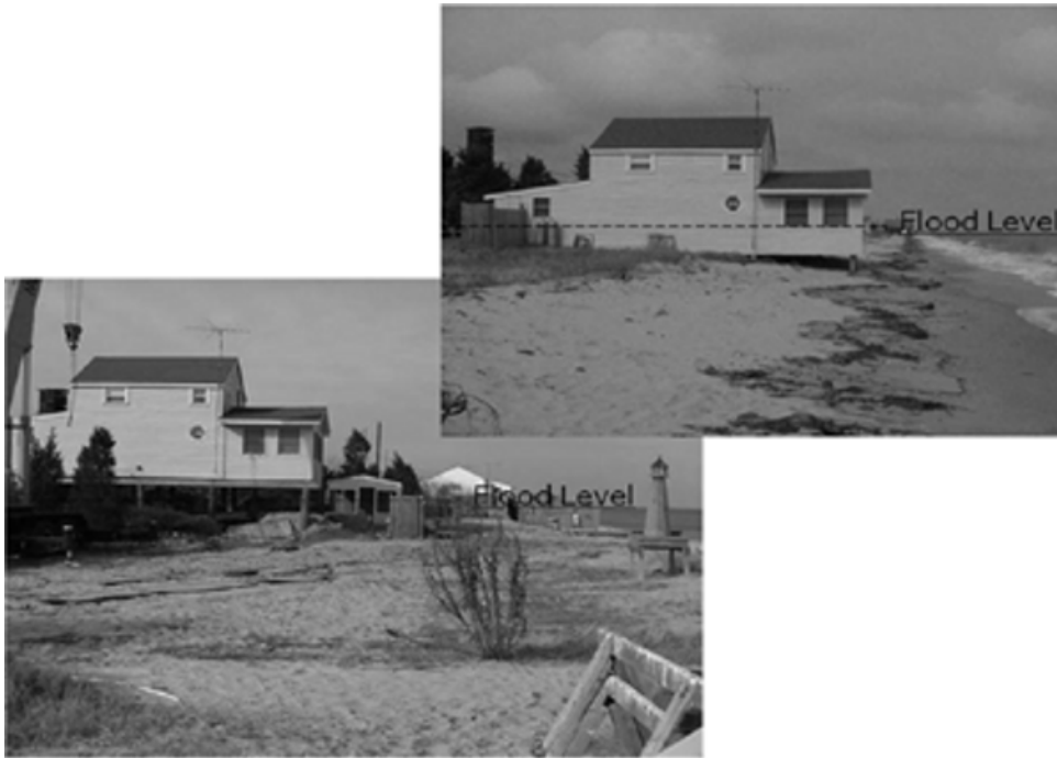
Figure 3: Elevation and relocation of a flood-prone home on the Delaware Bay.
